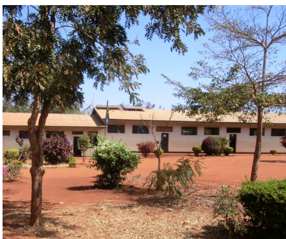
Figure 3: Solar power system installed at Banjika Secondary School (and other Schools under the Program).
