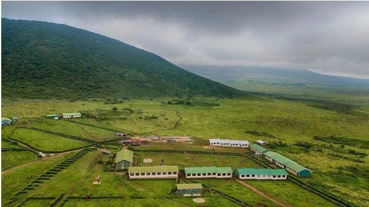
The Nainokanoka Secondary School in the Ngorongoro District, Tanzania, May 2018. (Photo: Powering Potential)
